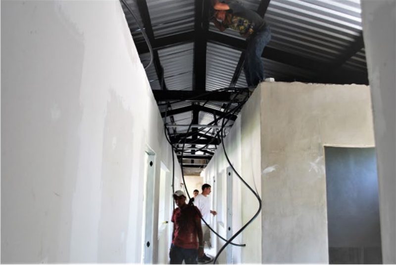
Finishing building the H2H clinic
