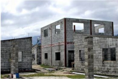
Boy's house under construction
